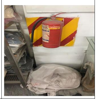
During site tour, it was noted the easy and un-obstructed access to one fire extinguisher was not provided in stitching section.
