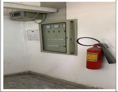
During factory tour, it was noted that Rubber sheet /Mat was not laid beneath the electric control panel near main gate.
